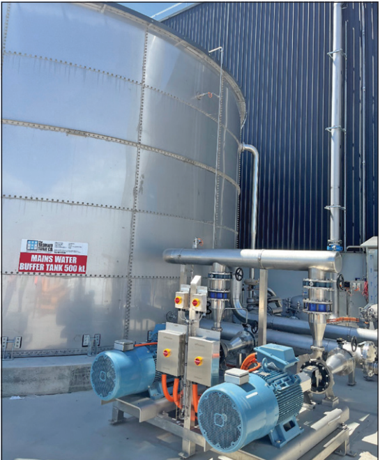
The on-site 500kL mains water buffer tank.
