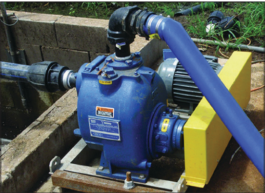
The Gorman-Rupp T2A3 B wastewater pump on site.
