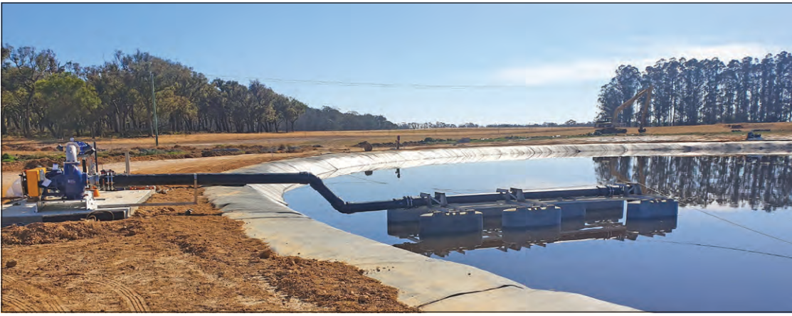
The Gorman-Rupp 86B3 self-priming pump securely mounted on the lagoon bank eliminates the need for workers to enter or operate directly on the water.
