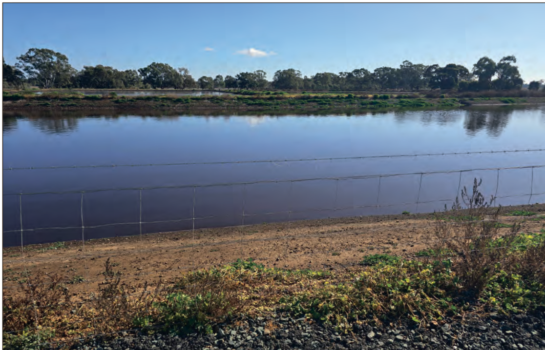
Early in the process, Scolexia undertook an effluent capacity assessment, confirming that the existing system could accommodate the return of pigs to the home farm.
