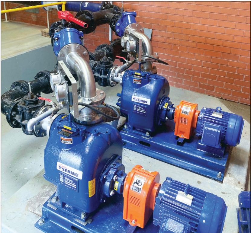
Wannon Water trialled the new technology, which has been in place for eight weeks without a single blockage, confirming the solids-handling capability of Gorman-Rupp's latest technology to handle extreme applications.
